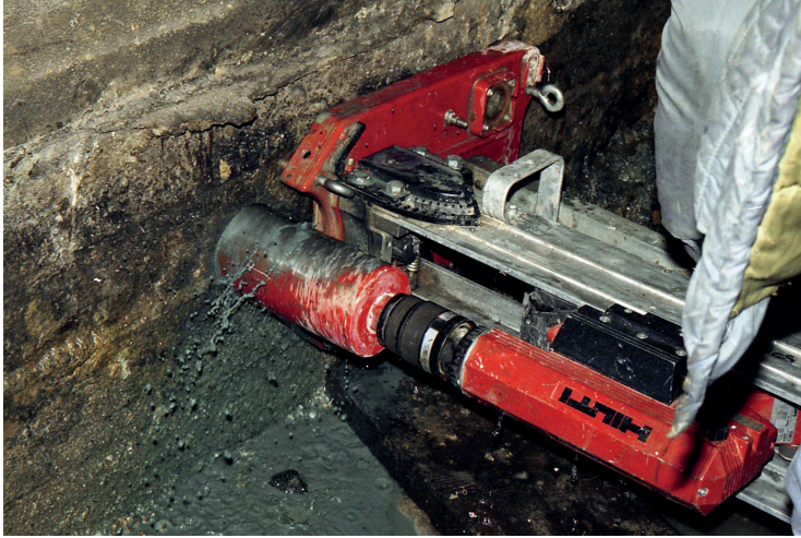
Fig. 3. Drilling the core no. 7 from the bottom plate of the foundation no. 1
