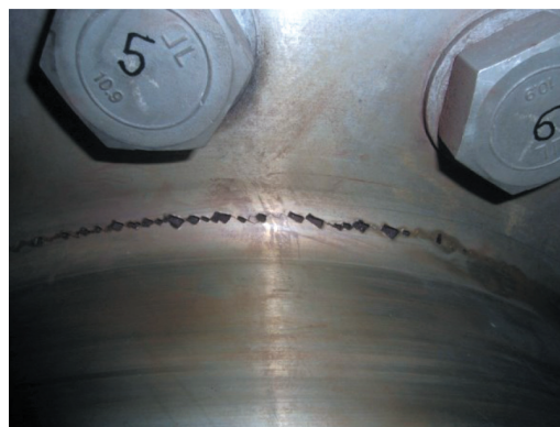
Fig. 2. Cracks in circumference with crushing [1]
